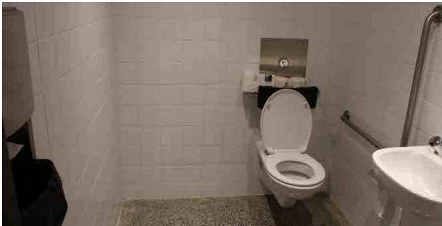
Image 12. Interior view of the men's accessible toilet
