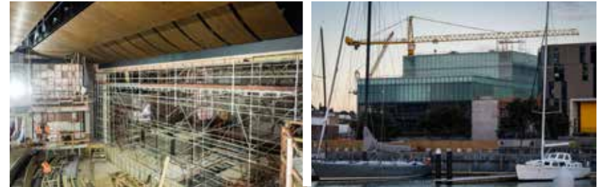
The ASB Waterfront Theatre stage and proscenium arch under construction.
